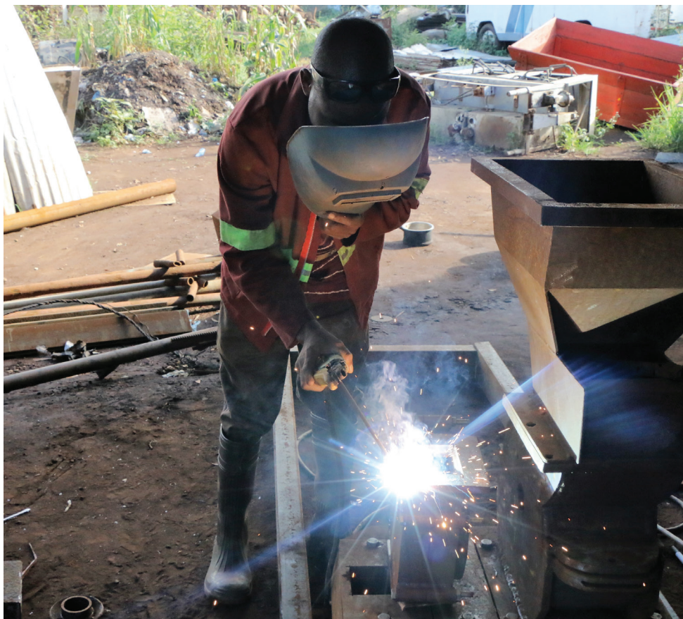
Small scale businesses rely on electricity for production
